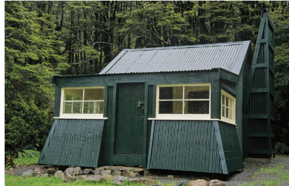
The restored roadman's hut, Jacks Hut, Arthur's Pass National Park, Canterbury, 2004. Built in 1879, it is a rare example of a roadman's cottage. It served as a bach for the Butler family for many decades from 1923. SHAUN BARNETT/BLACK ROBIN PHOTOGRAPHY
